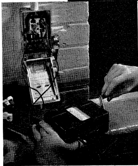
Figure 11 Making an insulation test at a switch-fuse
